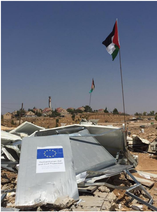
Demolished home in Umm al-Kher. Photo by Fadi Arouri. (See photo credits .)
